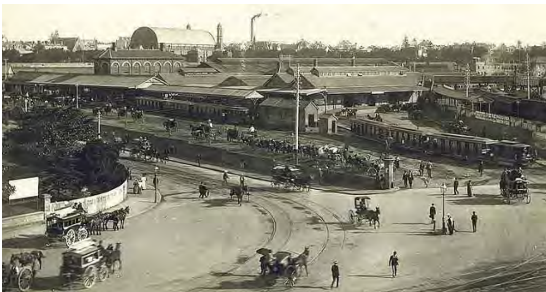
Figure 16 old Redfern (Sydney Terminus) Station SRNSW
