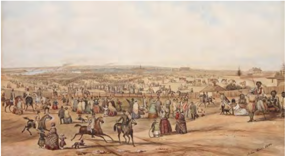
Figure 29 The turning of the first sod for the new railway station at Prince Alfred Park in July 1850, as depicted by John Rae, Mitchell Library, State Library of NSW - ML 244.
