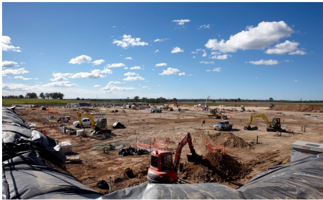
Work commences on stage one of the Oran Park Town Centre
